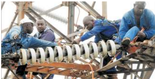
● Electricity engineers work on a power facility
