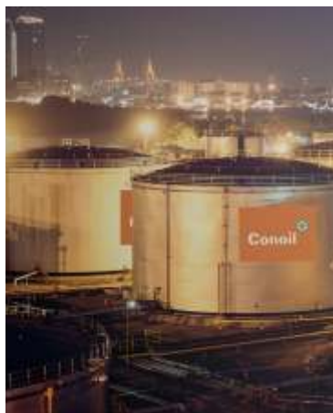
● Conoil tank farm
